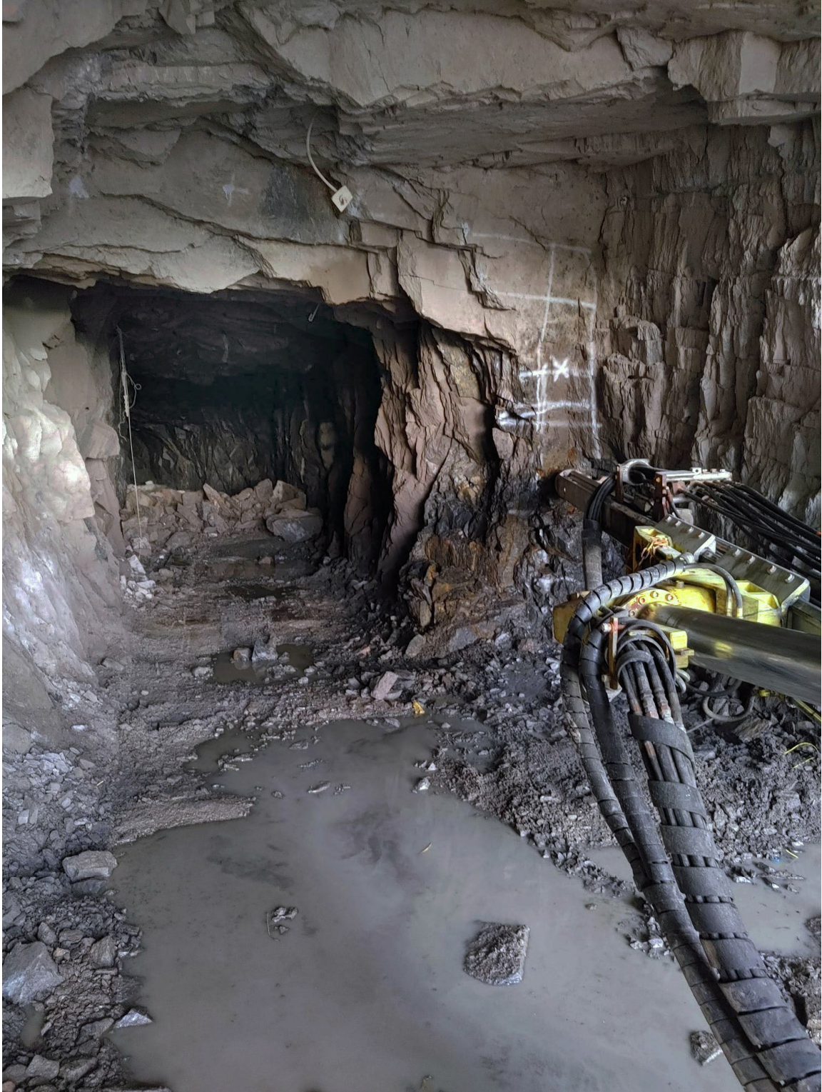
Photo 8. Slashing the historic workings to a 3m x 4 m size.
