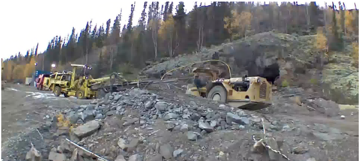
Photo 5. Electric hydraulic jumbo enroute to the ramp.
